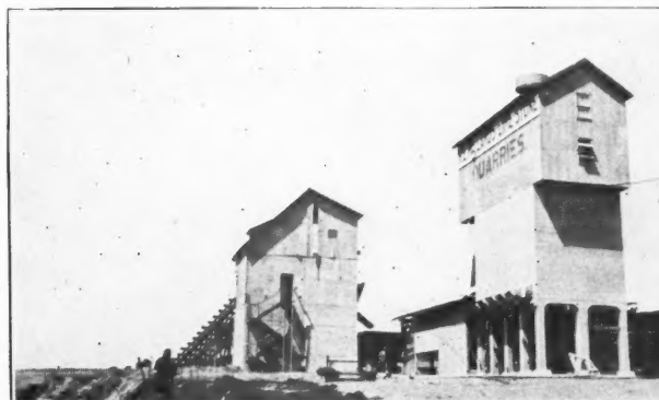
Hoist House at Left and Crushing Plant at Right
